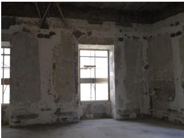
Office under refurbishment - 5 th floor
