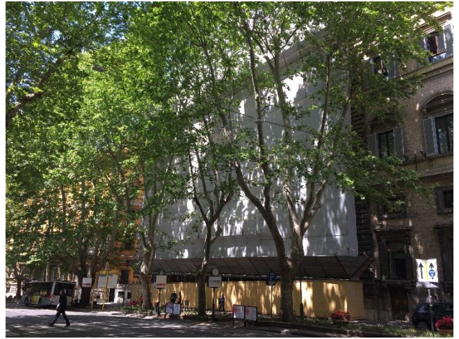
Main façade from Via V. Veneto
