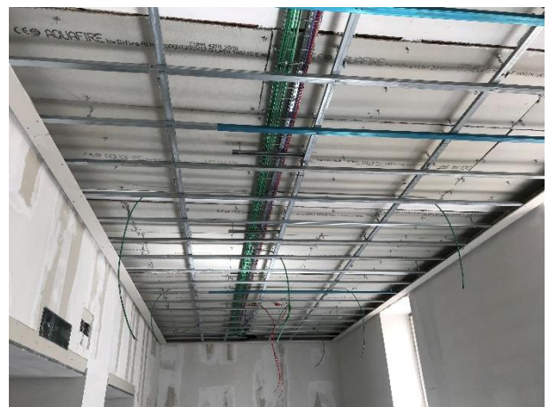
False ceiling on the Seventh Floor
