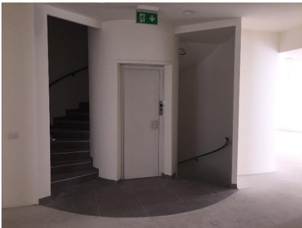
Access of the first floor
