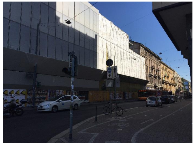
Façade along Via Padova
