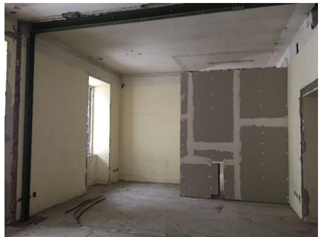
Interior (metal frame and new plasterboard partition)
