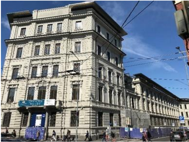
View of the building from Piazzale Lodi
