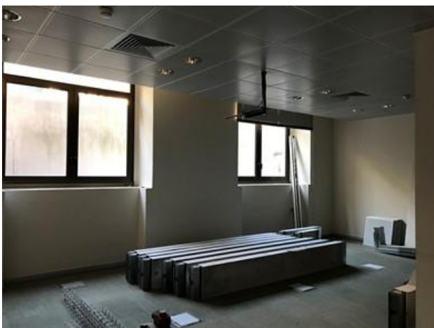
Offices on the basement floor
