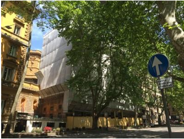
Main façade from Via V. Veneto
