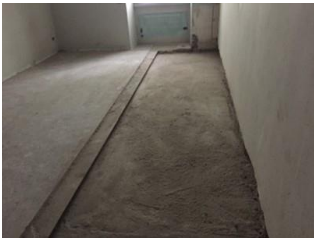
Interior (new portion of floor - 1 st floor)
