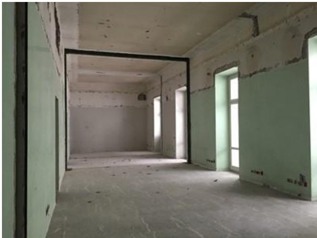
Office under refurbishment - 1 st floor
