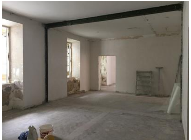
Office under refurbishment - 3 rd floor
