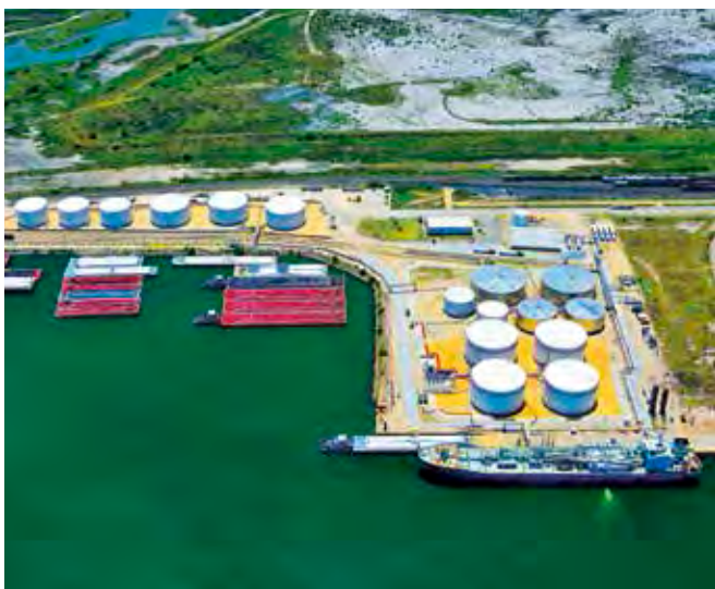
Oil storage terminal, Corpus Christi, Texas, US.
