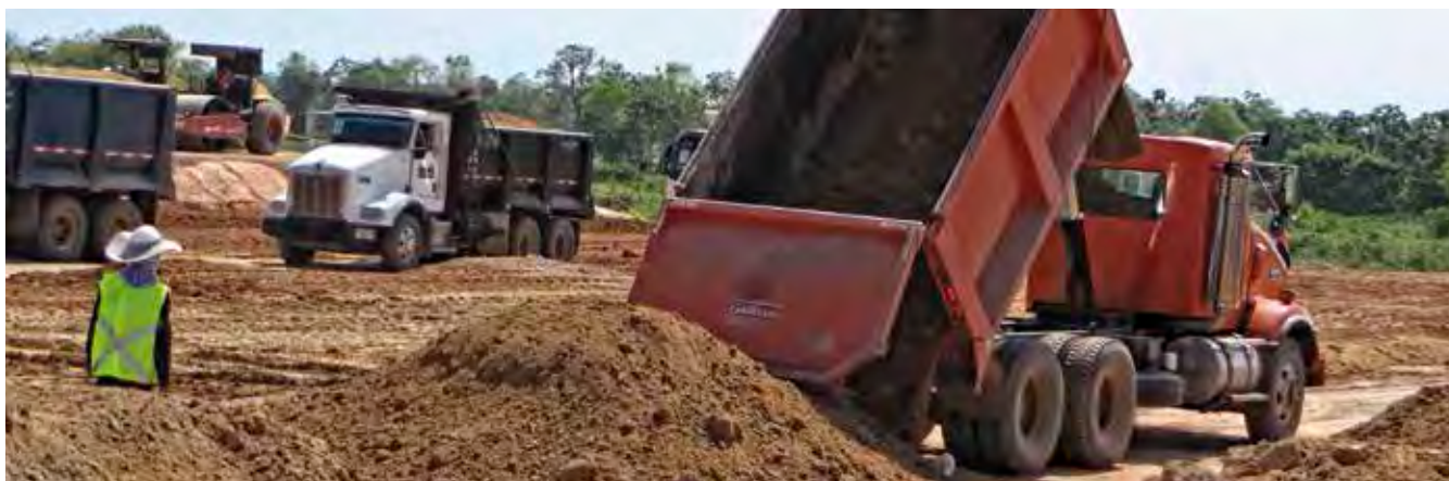
Construction of Impala Terminals' Barrancabermeja riverside port, Colombia.
